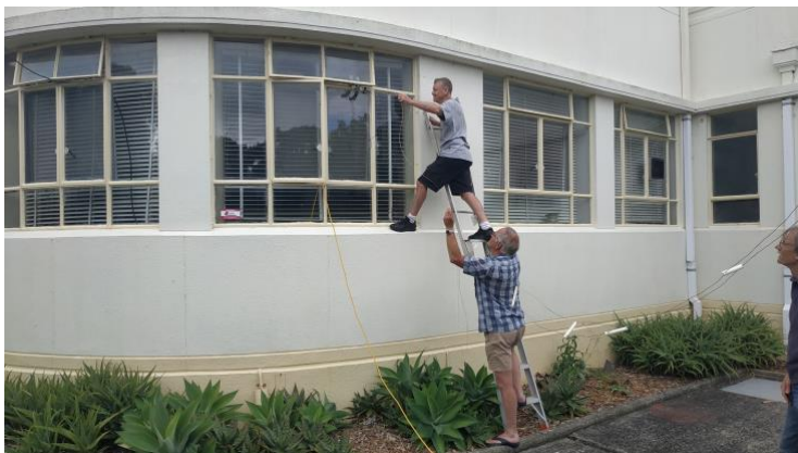
Forty meter twin lead repaired and threaded back through the 'temporary' feedthroughs- probably put up by Ian ZL1BFB (SK) in the 1990's. - Photos by ZL1DL.
