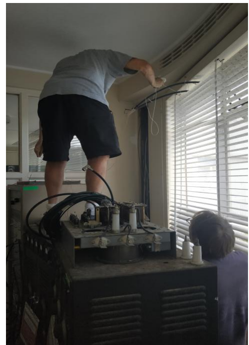
Forty meter twin lead repaired and threaded back through the 'temporary' feedthroughs- probably put up by Ian ZL1BFB (SK) in the 1990's. - Photos by ZL1DL.
